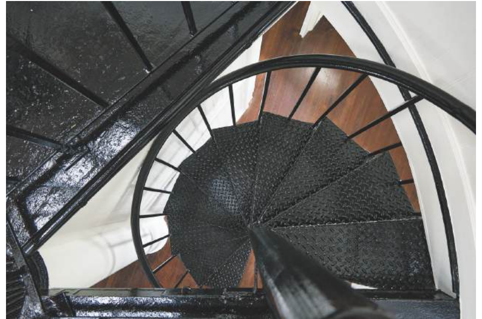
The spiral staircase between the fifth and sixth floors
